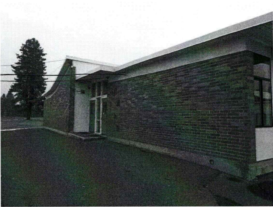
Figure 1: West Elevation of Building Area B
