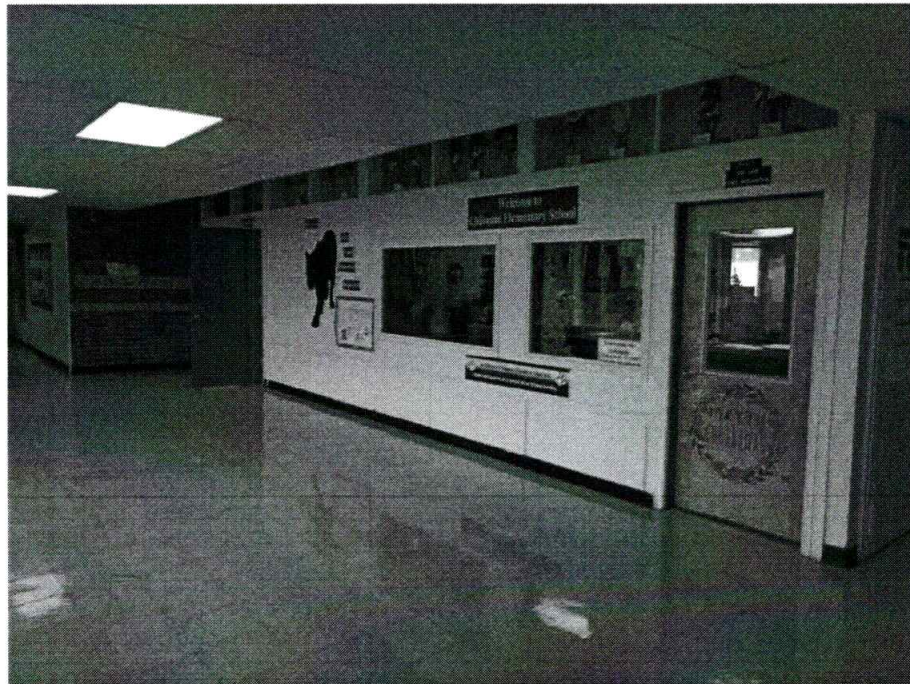
Figure 6: Interior Masonry Veneer
