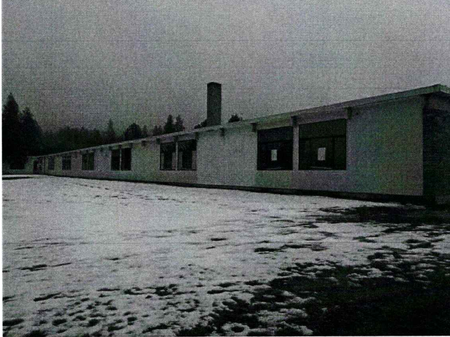
Figure 2: North Elevation of Building Area B
